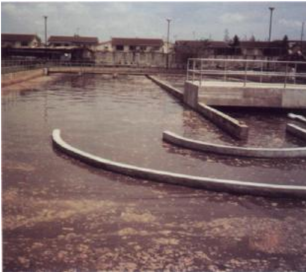
Effluent treatment plant in Hong Kong Fairview Park
