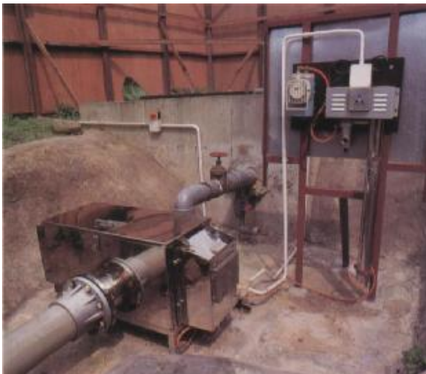
UV/Ozone system installed after the effluent treatment plant in a movie studio, for removal of color, bacteria and reduction of COD
